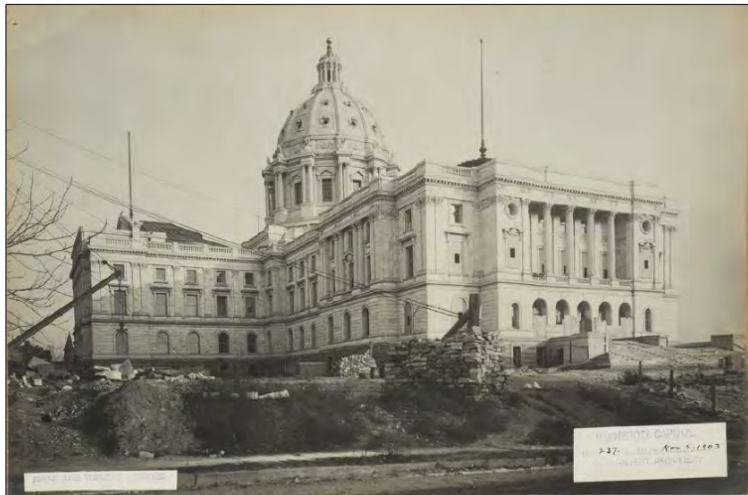
Capitol Building under Construction in 1903 108
