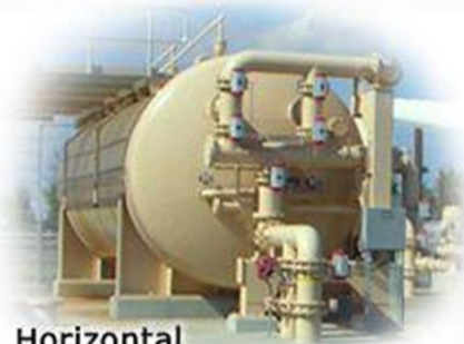
Horizontal Pressure Filter
