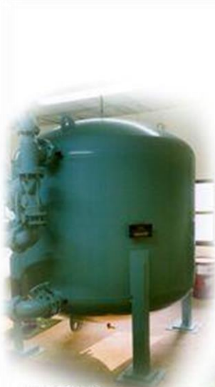
Vertical Pressure Filter
