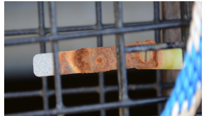
Tower 5 Control Tower
